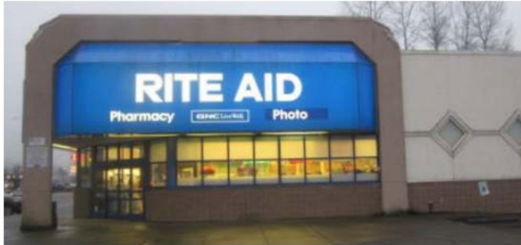
Remove and dispose of existing awning, patch penetrations with paintable sealant
