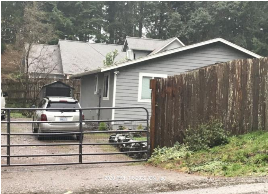
Figure 5: Photo dated 2020 shows front access and adjacent single-family residence to the west.
