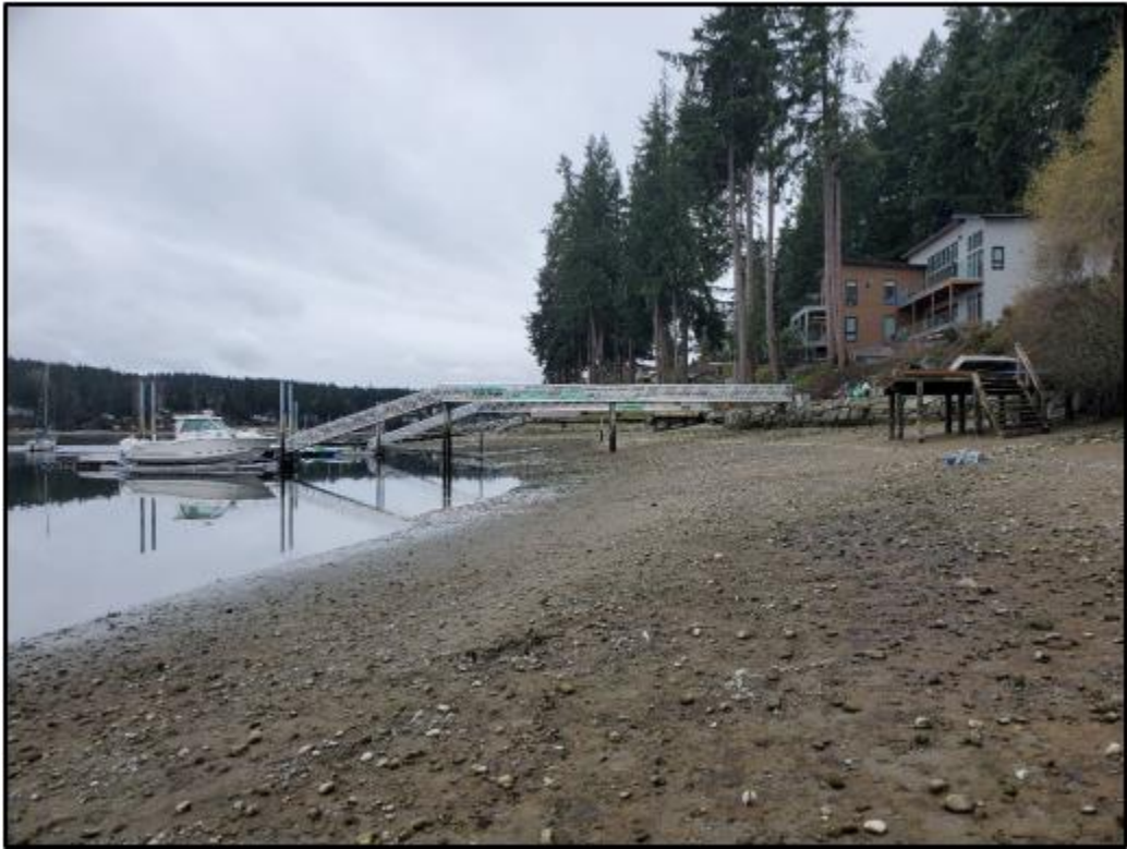
Looking south along the shoreline from the project area, along the shoreline.
