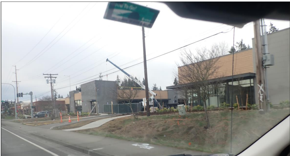
Photograph taken driving south on Meridian looking at the north and building elevation facing Meridian East.
