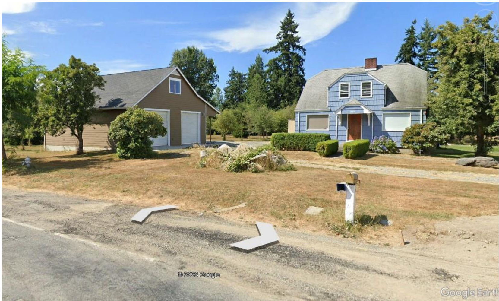
The barn and home from 85 th Street East (facing north) (Google Earth Image).
