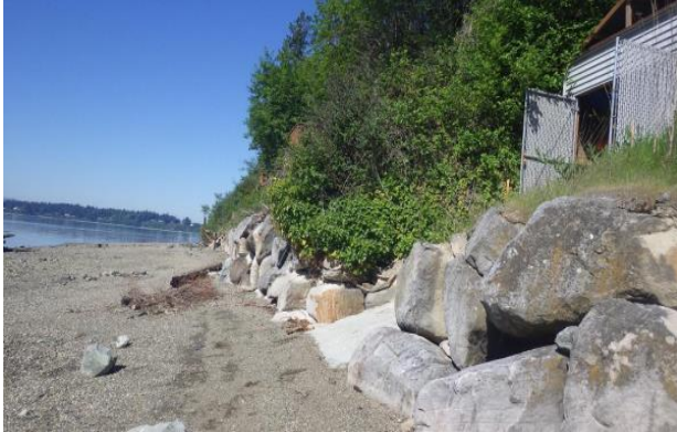
Looking NW at the Bulkhead
