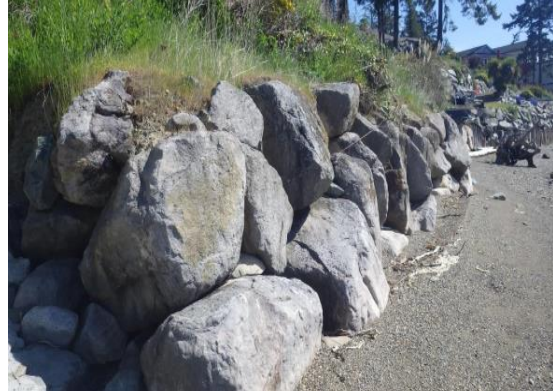
Looking SE at the Bulkhead
