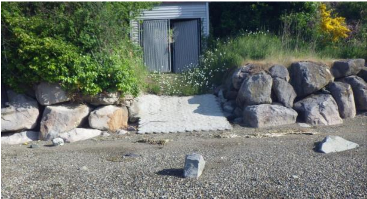
Existing boat ramp
