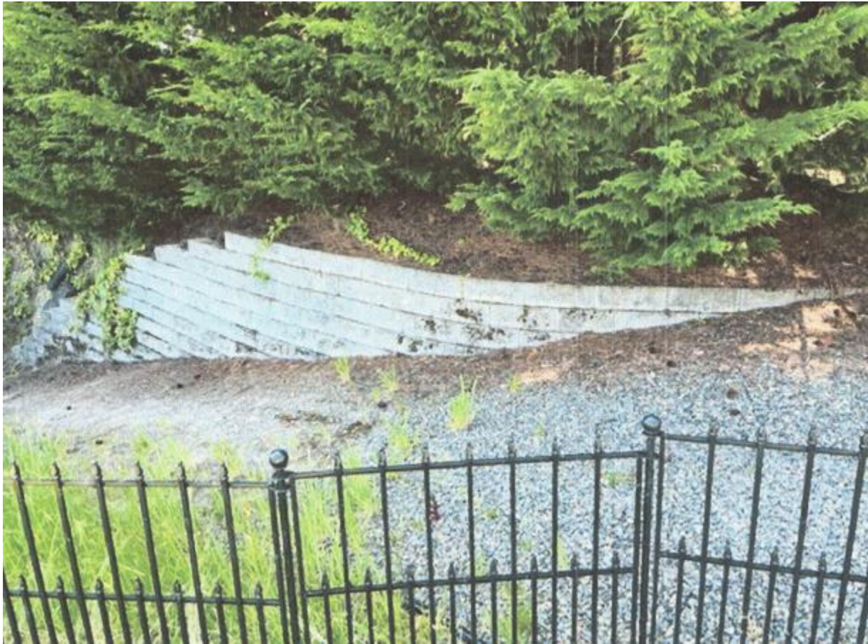
Exiting pathway and western retaining wall
