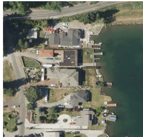
Figure 18S.20- 3 Example of Residential Shoreline Environment
